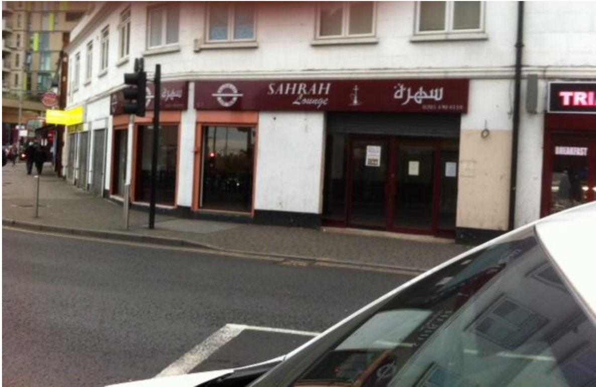
Image 2. View of front of premises from Wembley Hill Road
