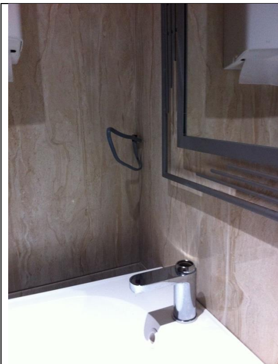
13 Exposed electrical cable next to wash hand basin in ladies WC
